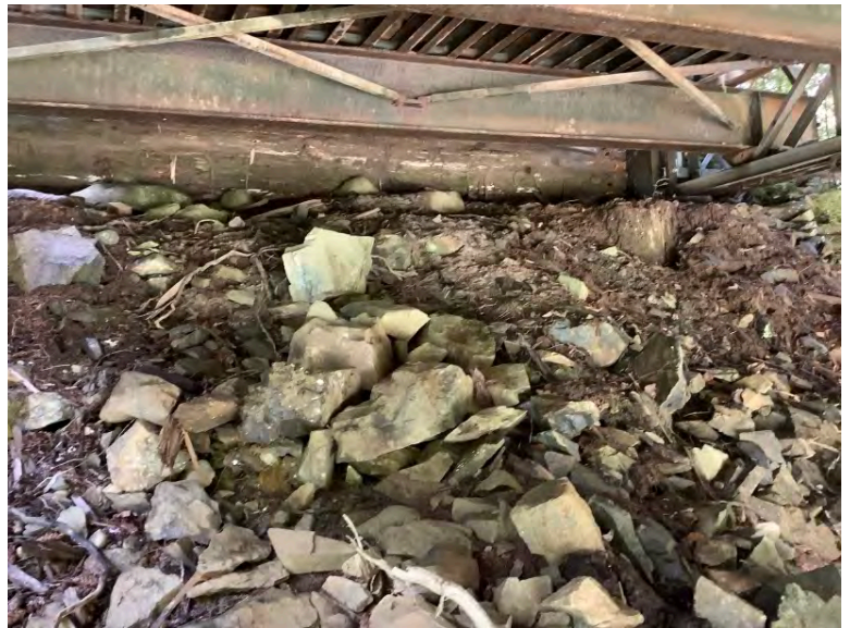
Right Bank Abutment when facing downstream
