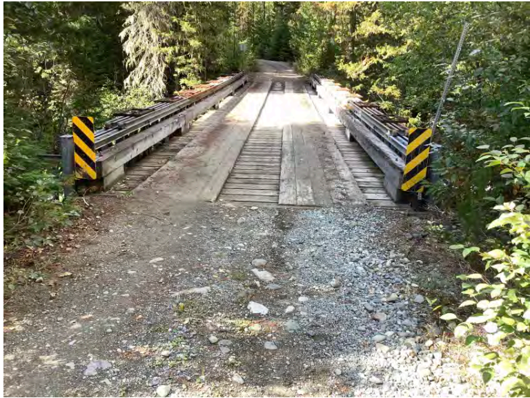
Approach from Left Bank when facing downstream
